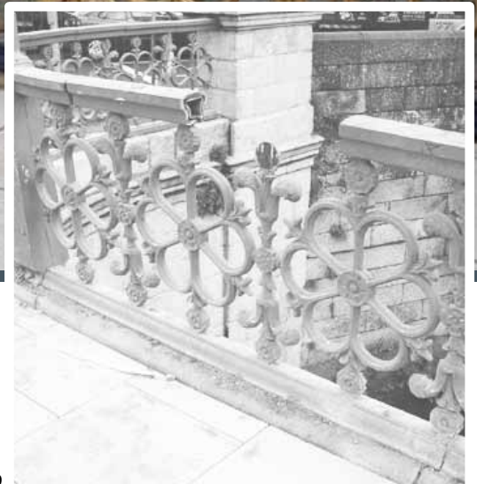
Pattern making and casting of replacement cast iron bridge railings. 2009
