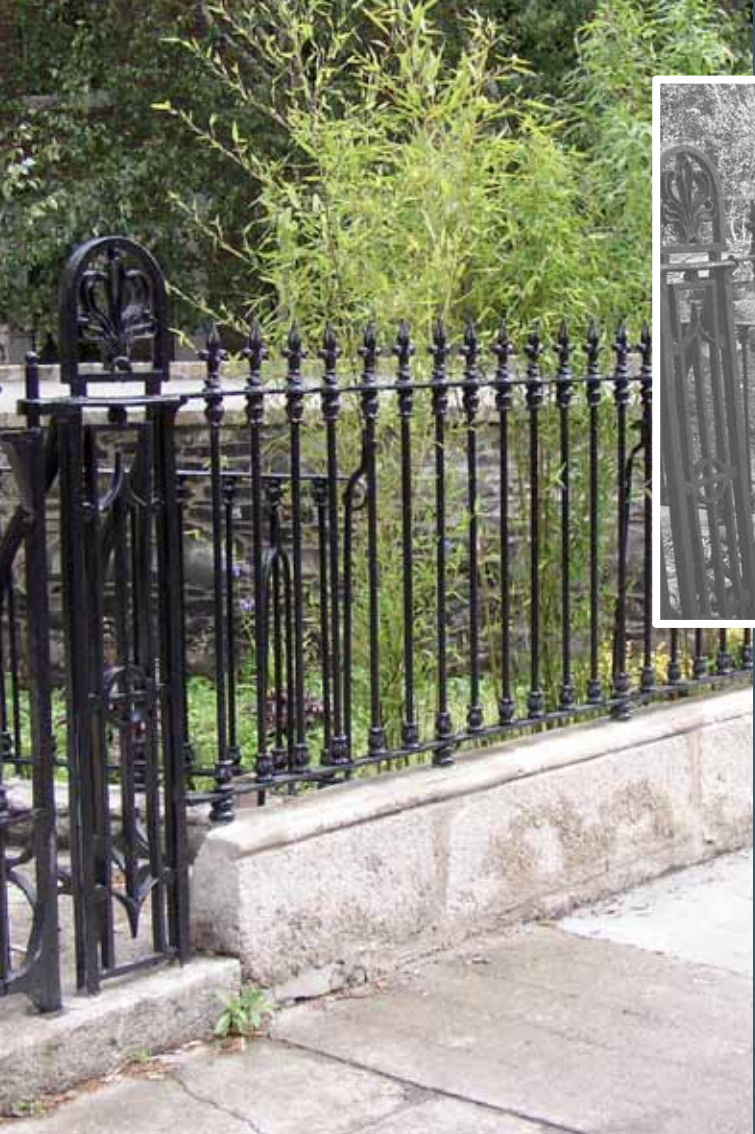
Restoration of 19th Century wrought and cast iron railings. 2010
