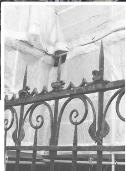
Restoration of wrought iron railings from Christchurch Cathedral dating from the 19th Century. 2009
